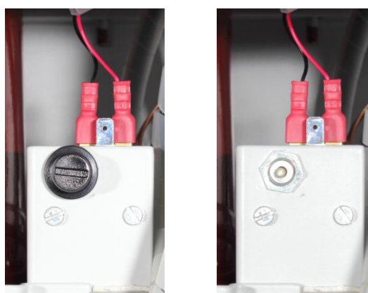
Fig. 4): Safety temperature limiter with (left) - and without protective cap (right)
